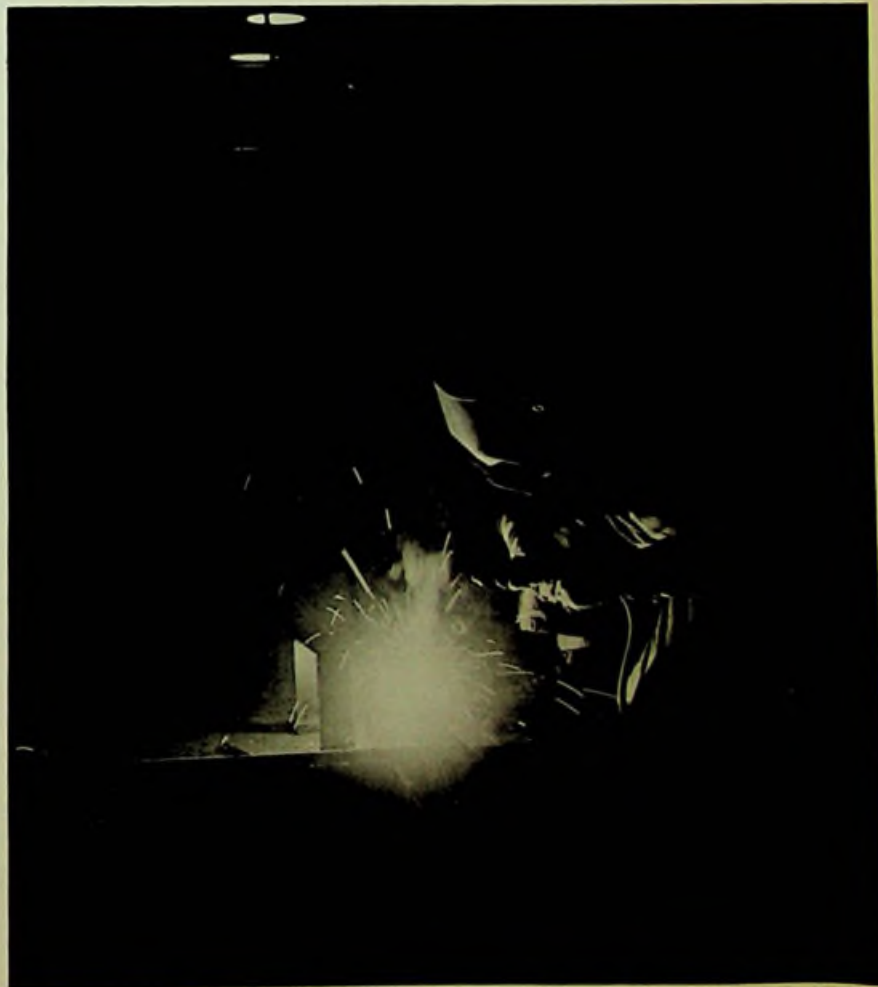
A member of the maintenance staff welds together the pieces of the damaged heating system.
